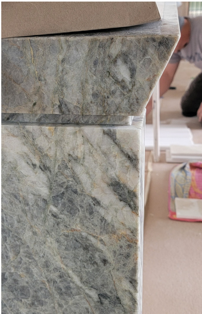
ANGLED MITERED EDGE WITH STONE REGLET DETAIL
